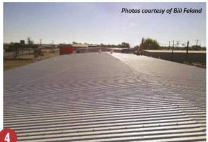
Metal roof after Rapid Roof® acrylic top-coat.
