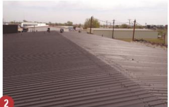
Metal after application of rust-inhibiting, Conklin Encase® Metal Primer.
