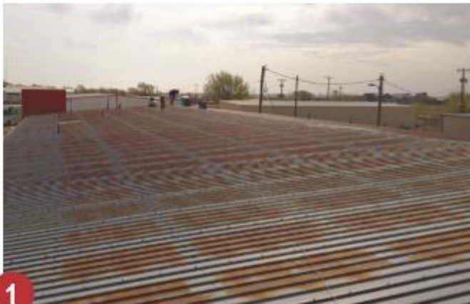
Rusty metal roof prior to restoration work.
